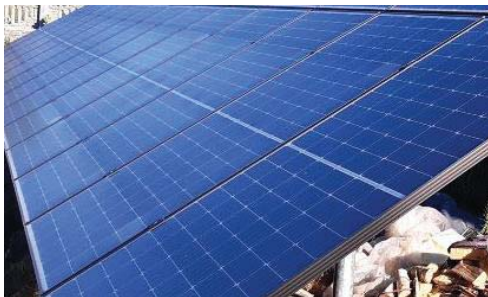
Figure 1. PV cell mounted in typical home power domain (author’s private PV system).
